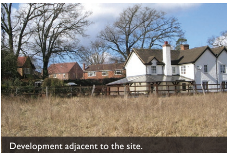
Development adjacent to the site.
